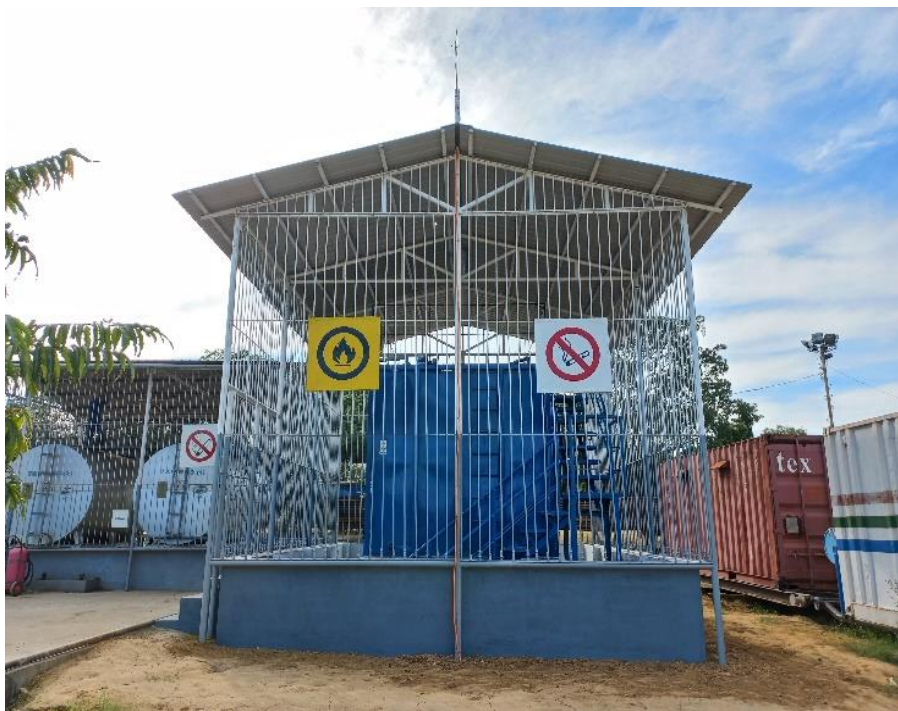
Figure 23: Containment of Diesel Storage Tank at Warehouse
