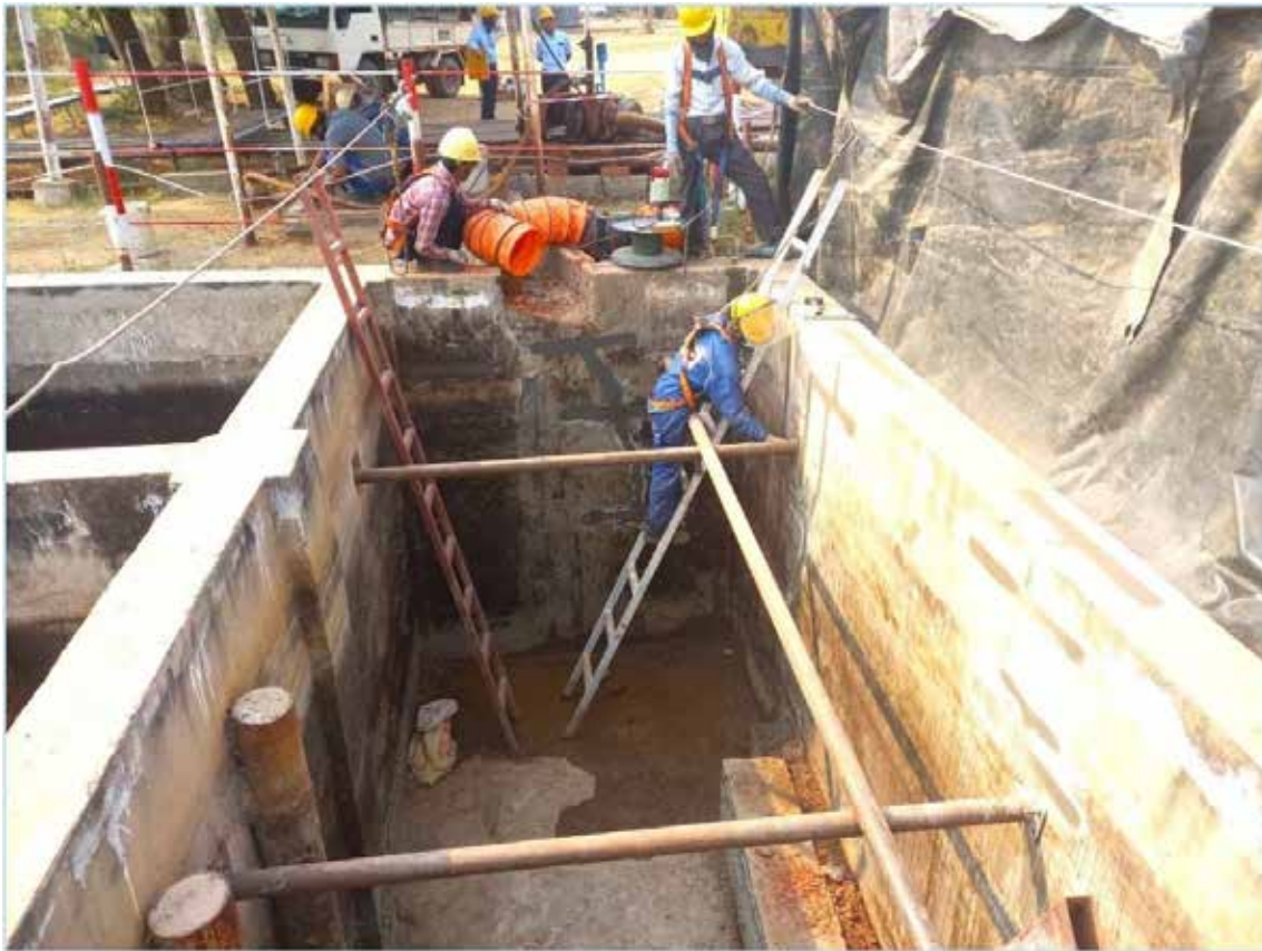
Figure 24: Produced Water Pit Repairing at GOCS-4
