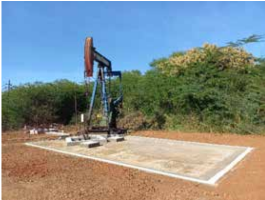
Figure 22: Constructed Concrete Pad and Additional Cellar at M-206
