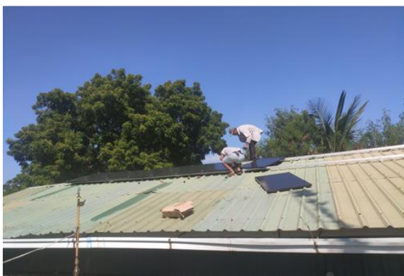
Figure 79: Installing Solar-Powered Water Pumping System at Aye Mya Village Existing Well
