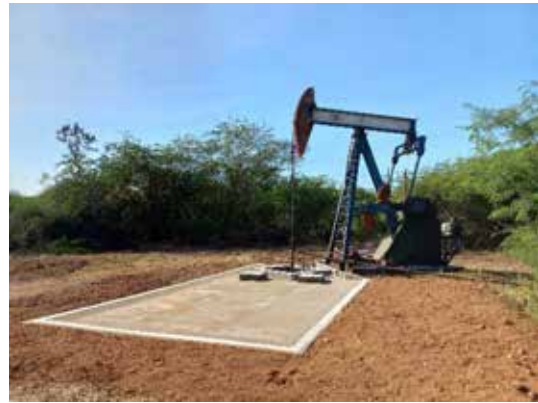
Figure 22: Constructed Concrete Pad and Additional Cellar at M-206
