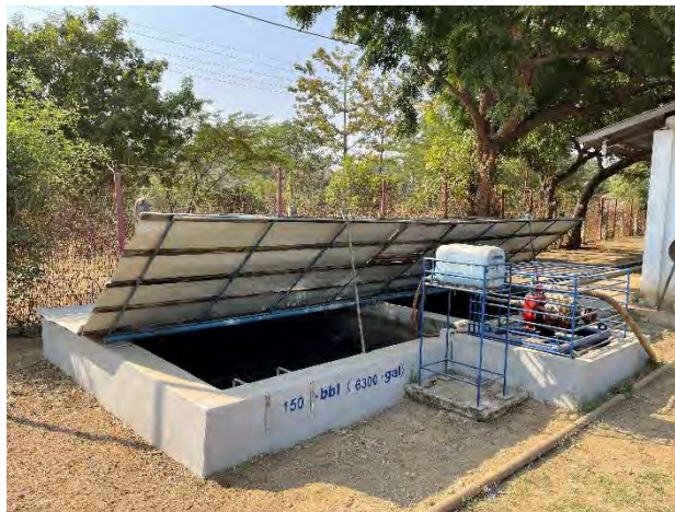
Figure 45: Warehouse Zero Discharge Tank
