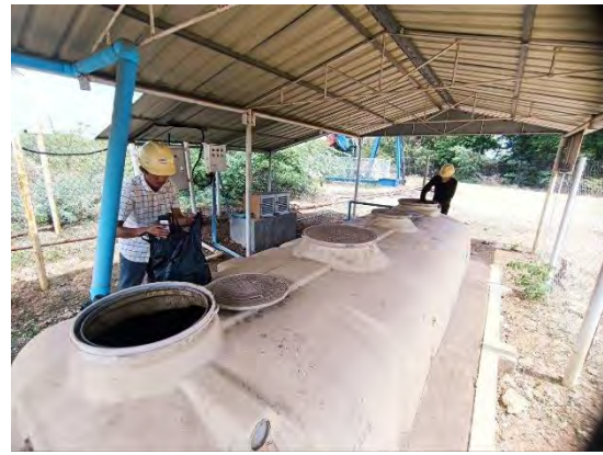
Figure 43: Regular Maintenance of Bio-filter by Third-party
