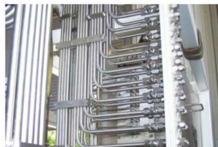
Fig. 3: Typical onshore hydraulic control unit (on left) with stainless steel tubing installed directly from the control unit to the valves or control devices (on right) (Source: Dynex/Rivett Inc)
