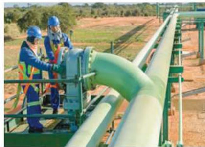
Fig. 7: Land vs deep-water pipeline crossing, a simple surface 16" pipeline tee (or T-crossing) is replaced with a massive subsea Inline Tee (ILT) (Source: gasprocessingnews.com and EAB Engineering)
