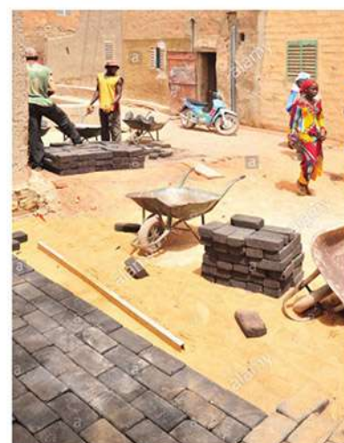
Fig. 6: Paving stones from plastics garbage and sand in Mopti (Mali, West Africa)
