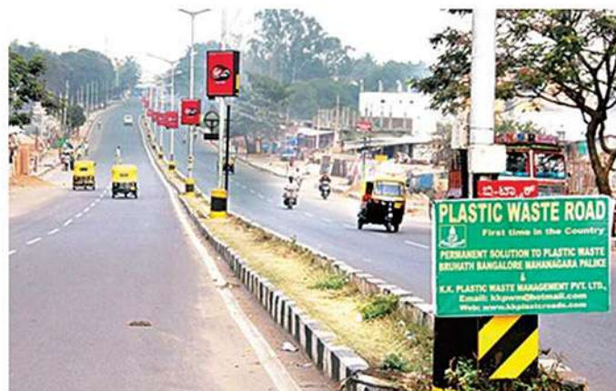
Fig. 5: A road in India made of plastic waste
