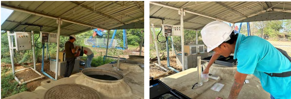
Figure 45: Regular Maintenance of Bio-filter by Third-party
