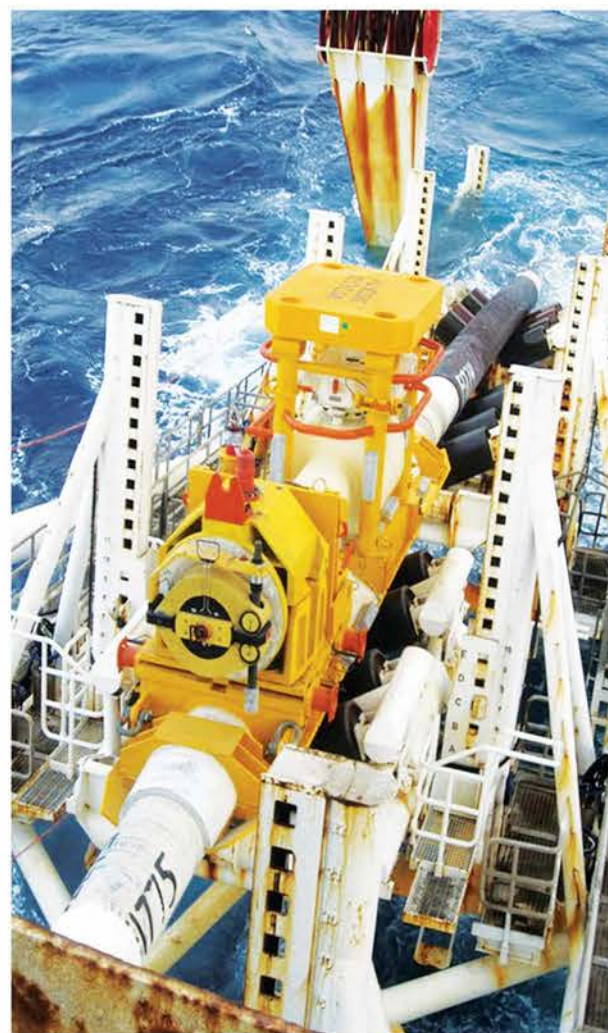
In-Line Tee (ILT) during flowline installation
