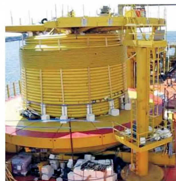
Umbilical loaded onto an Installation Carousel, preparing for installation by the installation vessel
