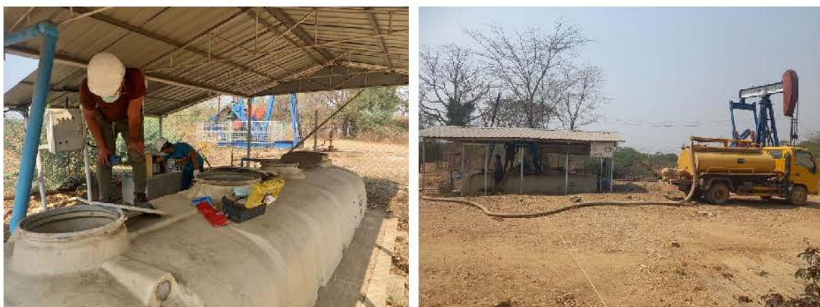
Figure 39: Desludging and third-party regular maintenance of Bio-Filter
