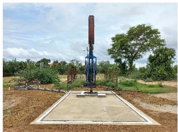
Figure 22: Concrete pad and additional cellar at M-16 and M-80
