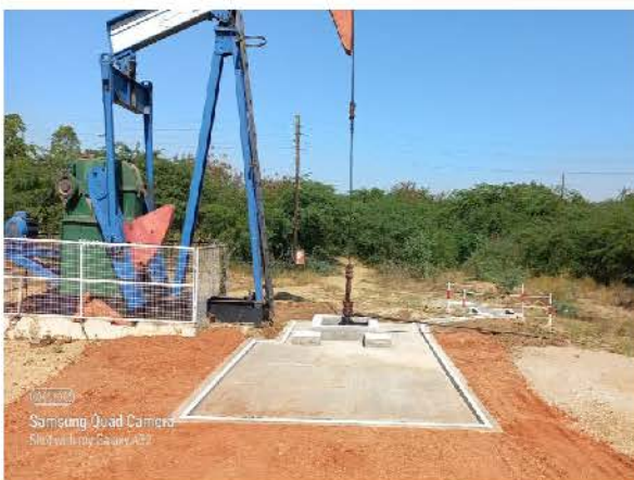
Figure 22: Concrete pad and additional cellar at M-16 and M-80
