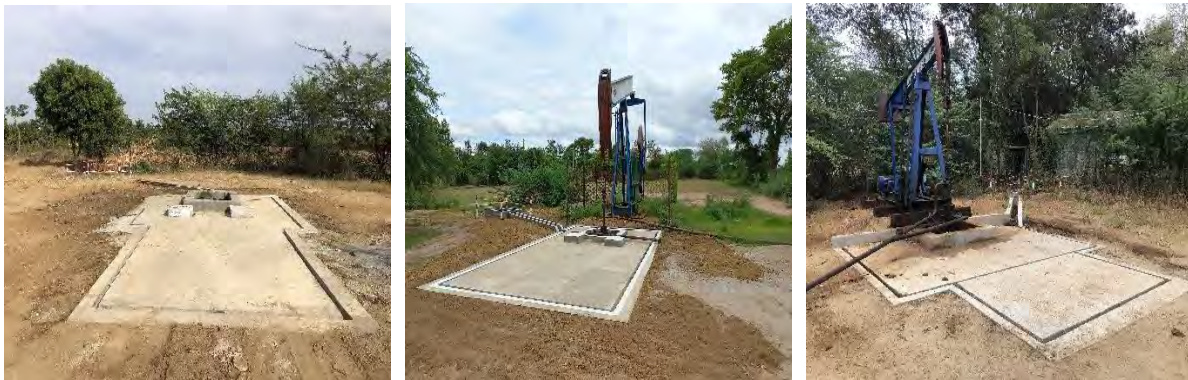
Figure 4: Concrete Pad and Additional Cellars at M-290, M-80 & M-554
