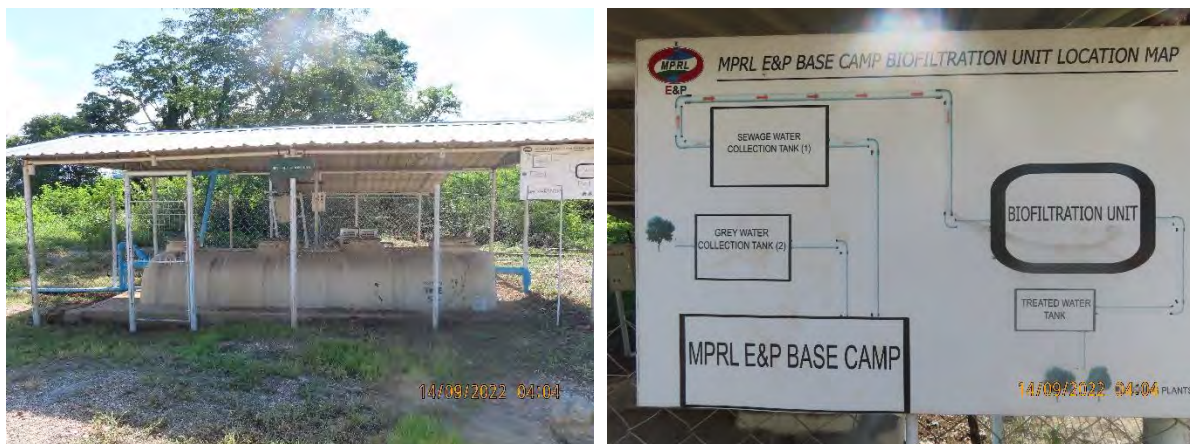
Figure 32: Bio-Filter Treatment System at MFO
