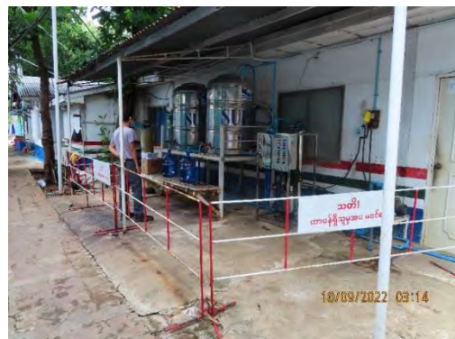
Figure 37: Reverse Osmosis (RO) Treatment System at Base Camp
