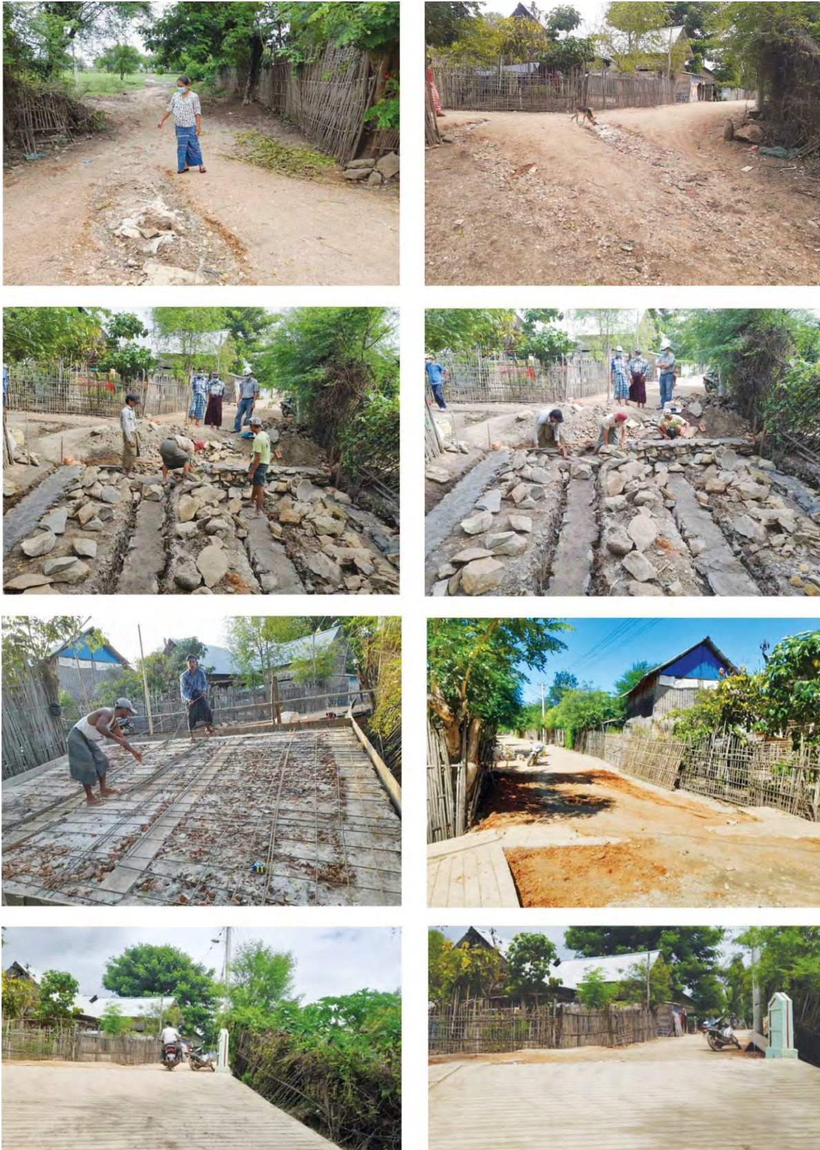
Figure 73: Provision of Road Concrete Slab and Drainage Construction in Mann Kyoe Village
