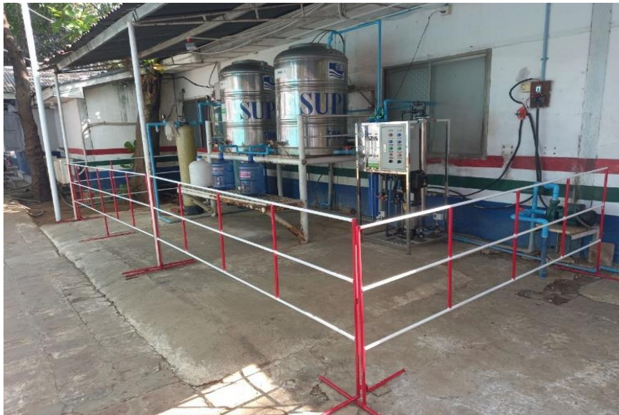
Figure 32: Reverse Osmosis (RO) Treatment at Base Camp
