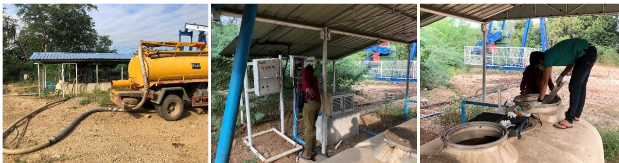
Figure 27: Maintenance Service at Bio filter Treatment
