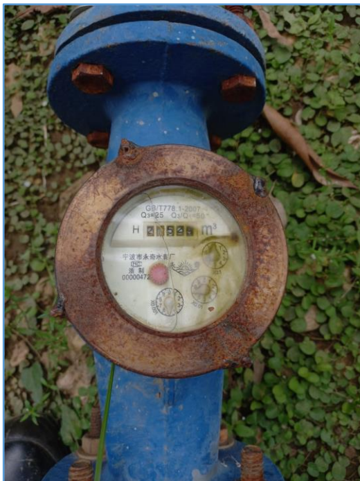
Figure 44: Monitoring with Water Flow Meter
