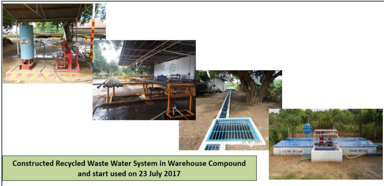
Figure 52: Recycle Water Usage System with Zero Discharge
