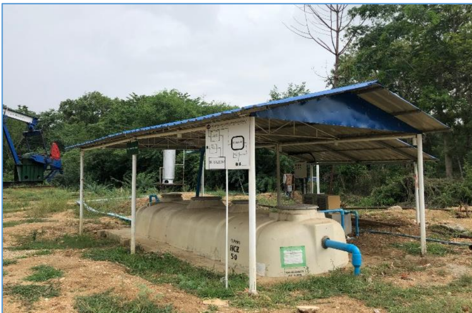
Figure 46: Bio-Filtration Unit
