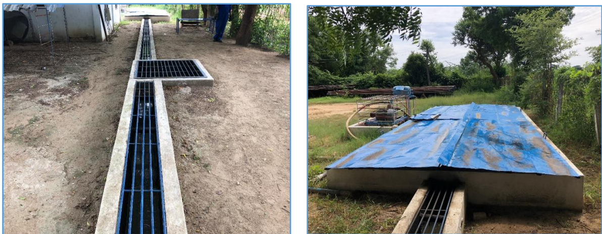
Figure 53: Recycle Water Back to Main Storage Concrete Pit
