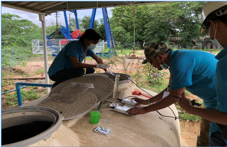
Performing maintenance and inspection for Bio filtration unit by authorized person from WM Water Company.
