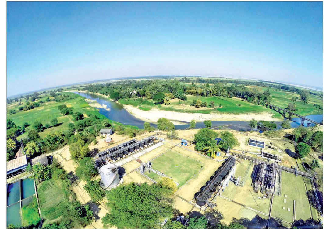
Aerial View of Mann Field Project located in Minbu, Magwe Region, Central Myanmar
